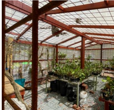
The secure new orchid house in the plant nursery area.
